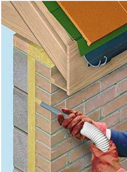
Poliuretano espanso in loco ( \lambda = 0.03 \text{ W/mK} )
